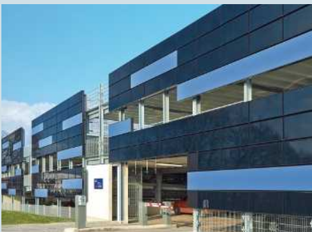
Building-integrated photovoltaics (BIPV)
