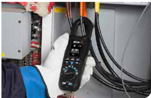
Verify amperage measurements
