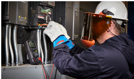
Troubleshoot Variable Frequency Drives using VFD mode
