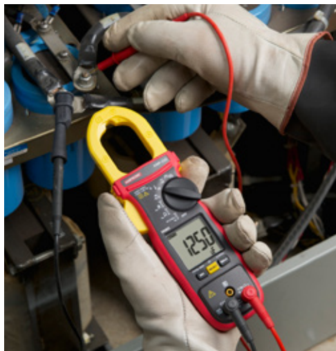
AMP-320 AC/DC Clamp Meter Electrical Motor Maintenance
