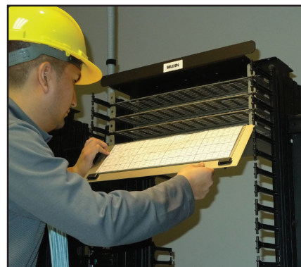
Shelf identification labeling is clearly visible.
