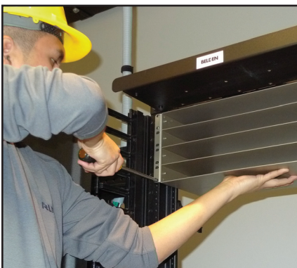
A single installer can install the system.
